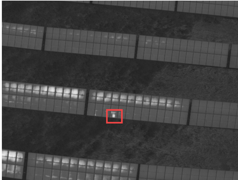
Thermal drone image
